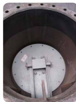
风机出口压力调节阀 Automatic pressure regulating valve
