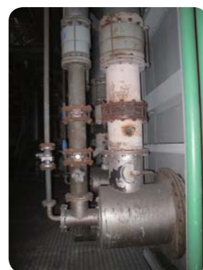
混合煤气调焰烧嘴 Mixed gas flame-adjusting burners
